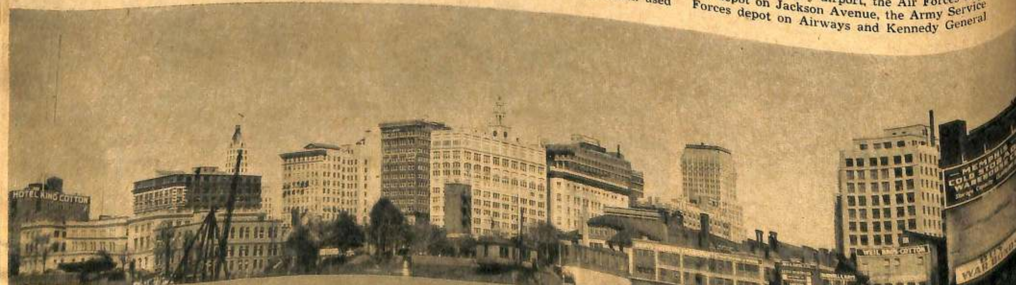
A skyline view of Memphis from the Mississippi. Warehouses line the river's edge and in the background is the business district with tall buildings.
