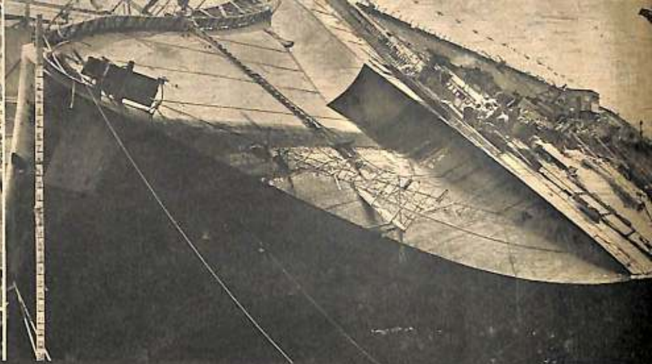
Tests proved the hull to be watertight in July and raising began Aug. 5. A week later the vessel had lifted from 79 to 36 degrees, was moving toward the desired 30.
