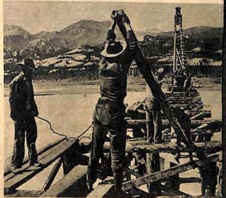
U.S. Army Engineers build bridge linking highway.
