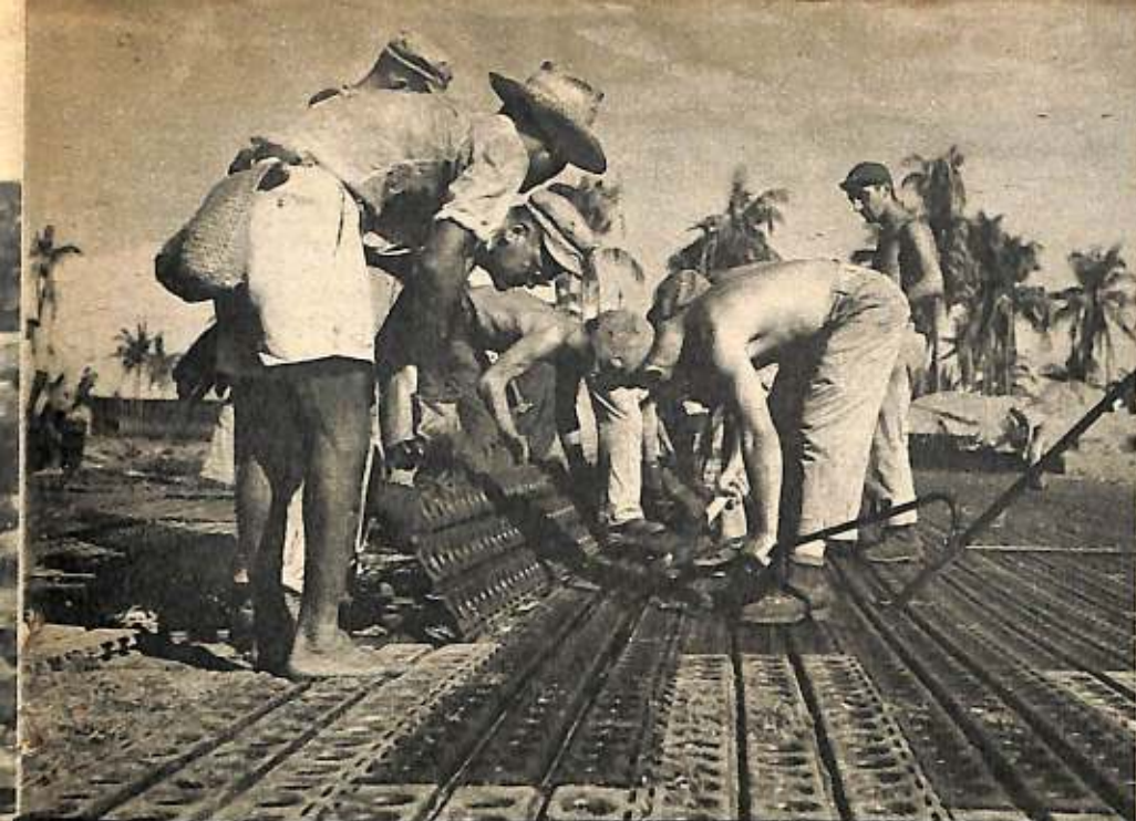
FILIPINOS HELP THE ARMY BUILD ROADS, BRIDGES AND AIRFIELDS. THE NATIVE AT THE LEFT LENDS A HAND TO GI ENGINEERS LAYING A SECTION OF MATTING ON AN AIRSTRIP.
