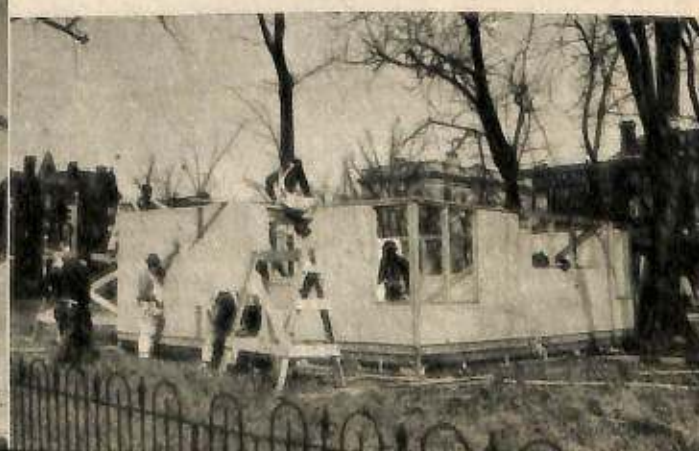
HOME ABROAD. WORKMEN IN WASHINGTON, D. C., PUT TOGETHER A DISPLAY MODEL OF THE 30,000 PREFABRICATED HOUSES TO BE SENT TO SHELTER BRITAIN'S BLITZED HOMELESS.
