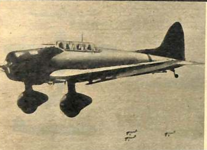
"VAL." Jap dive-bomber made by Aichi who, having left the landing gear sticking down, has produced a plane easily spotted. Val can't pull its landing gear up. It has a long fin faired into the fuselage, elliptical wings, diving brakes, a high Jap greenhouse and a sharp taper to leading edge of stabilizer.
