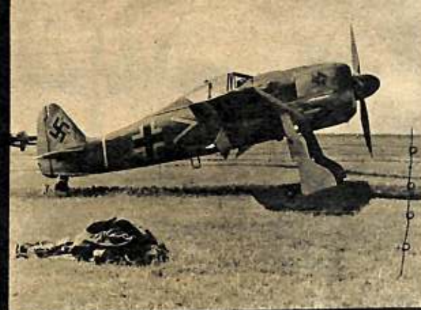
FW-190. This is the only German single-engine fighter with a radial engine. Because both the Focke-Wulf job and our P-47 have radials, they may be confused. In head-on view FW-190 has fuselage on top of wing, while P-47's belly bulges below wing. Tails also differ, FW-190's being thin and square.
