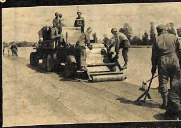
5 A TRACTOR AND CARRY-ALL "SKINS THE SOD" TO REMOVE THE OVERWORKED AND SPONGY TOP SURFACE.
