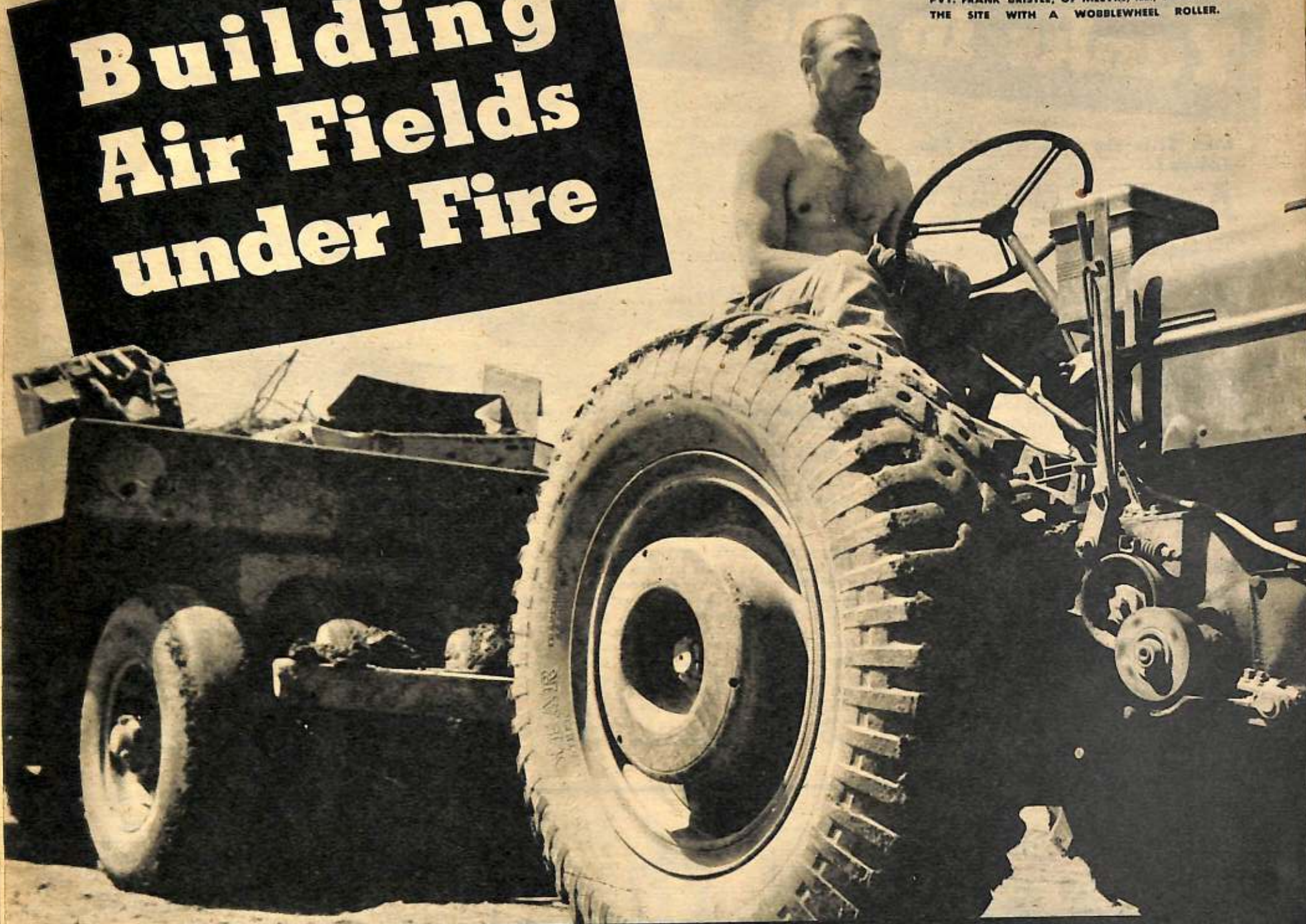
PVT. FRANK BRISTLE, OF MELVIN, ILL., SMOOTHS THE SITE WITH A WOBBLEWHEEL ROLLER.
