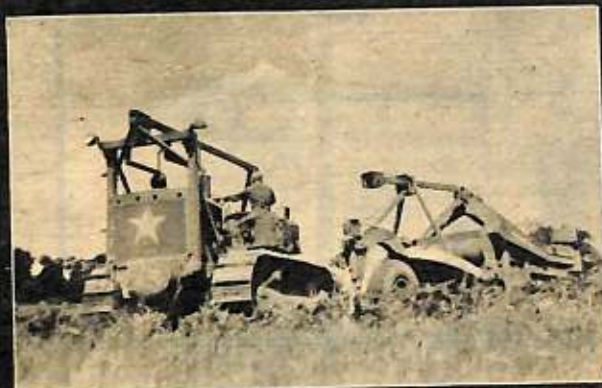
5 A TRACTOR AND CARRY-ALL "SKINS THE SOD" TO REMOVE THE OVERWORKED AND SPONGY TOP SURFACE.
