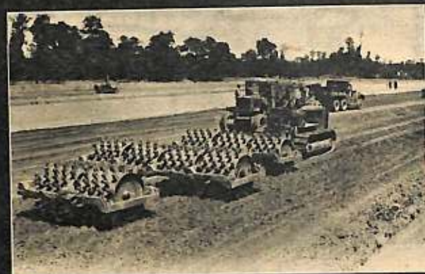
6 CARRY-ALLS, GRADERS, ROLLERS, AND WATER SPRINKLERS SQUASH THE SOIL INTO BRICK-LIKE HARDNESS.
