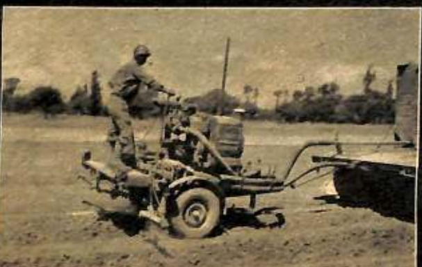
7 T/5 JOHN J. PARISE, EX-TRUCKER FROM PORT RICHMOND, N. Y., RUNS THE NINTH'S WATER-SPRINKLER.
