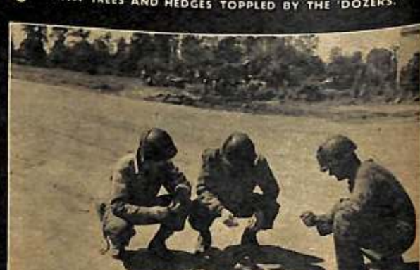
9 ENGINEERS EXAMINE THE TOP SURFACE TO MAKE SURE LANDING MATS CAN BE SECURELY LAYED IN PLACE.
