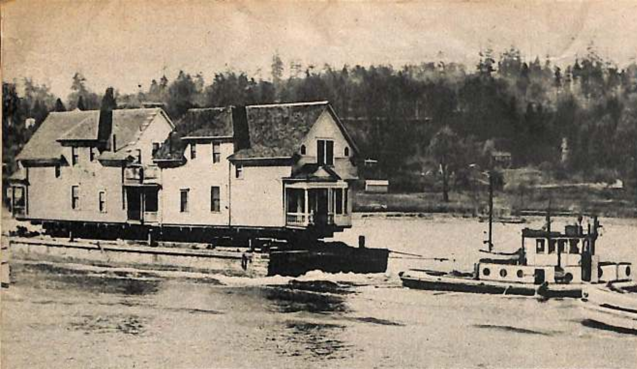
WATER MOVE. THE HOUSING SHORTAGE IS SO ACUTE IN SEATTLE THAT THEY DON'T TEAR DOWN OLD HOUSES TO MAKE WAY FOR NEW ONES. THEY JUST BARGE THE OLD-TIMERS VIA PUGET SOUND TO WHERE THEY'RE NEEDED.
