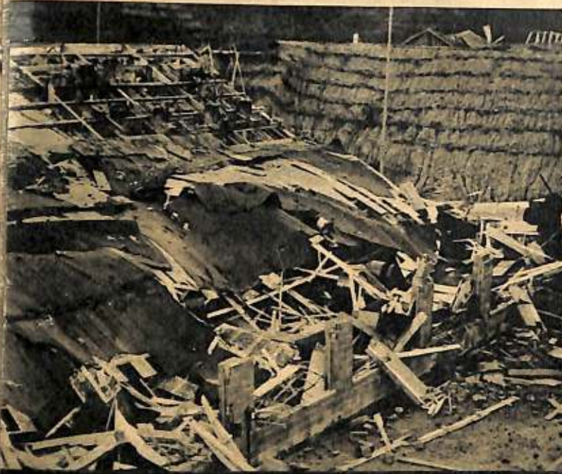
This wreckage is all that was left of some of the buildings blown up in an explosion at the Navy Mine Depot, Yorktown, Va. Six civilian workers were killed and 20 were injured.
