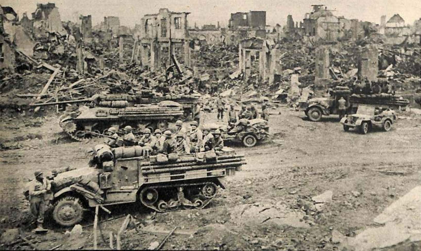
AS SOON AS DUREN HAD FALLEN TO THE FIRST ARMY DOUGHBOYS PUSHING ACROSS THE ROER, IT BECAME THE JUMPING-OFF PLACE FOR NEW ALLIED DRIVES TOWARD THE RHINE. THE ENGINEERS GREW MORE HAIR ON THEIR EARS DURING THE CROSSING, BUT (ABOVE) THEY GET READY TO ADVANCE AGAIN.
