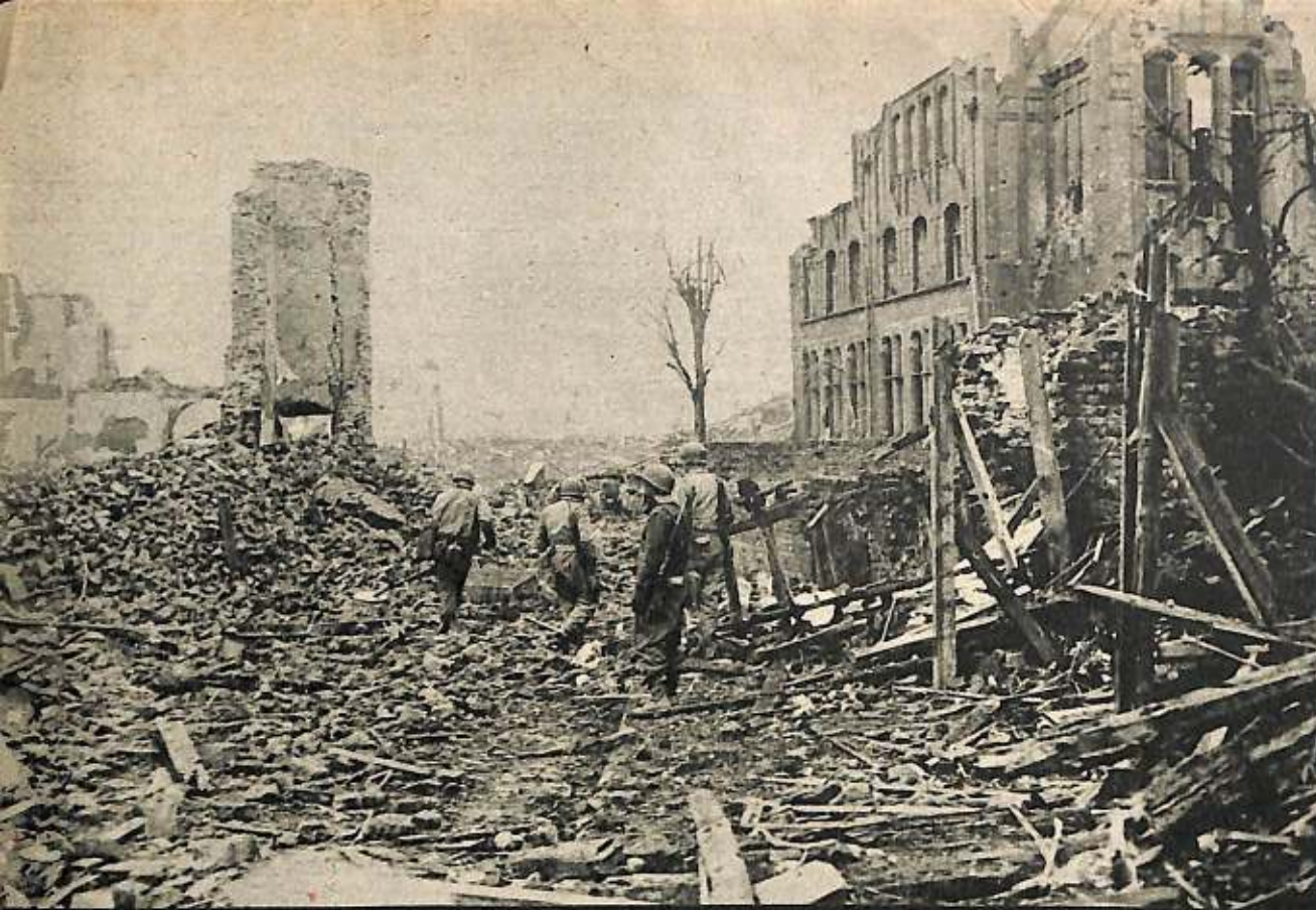
THIS MINE-SWEEPING PATROL OF THE 8TH DIVISION ADVANCES AHEAD OF INFANTRY UNITS TO SWEEP A SAFE PATH THROUGH THE RUBBLE THAT WAS ONCE DUREN. THE CITY WAS CLEARED OF ENEMY FORCES FEB. 25, 1945.
