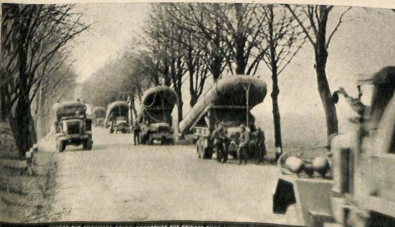
BEFORE THE ENGINEERS COULD CONSTRUCT THE BRIDGES THAT CARRIED HEAVY EQUIPMENT ACROSS THE ROER, THE HUGE RUBBER PONTOONS HAD TO BE BROUGHT UP FROM THE REAR. HERE THE DRIVERS ARE ABOUT TO BEGIN THE LAST LAP.
