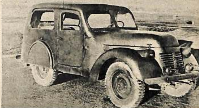
AND THIS IS A JEEP THAT HAS BEEN BUSTED TO A CIVILIAN. MEN AT AN 8TH AAF BOMBER STATION USED ONLY SALVAGED MATERIAL IN KNOCKING TOGETHER THIS STREAMLINED PEACETIME VERSION OF THE OLD WORKHORSE.
