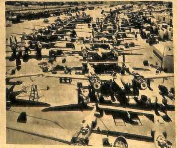
At Burbank, Calif., Lockheed Lightnings get a final going over by assembly workers out of doors. The P-38s were assembled outside of the plant during a switch-over to a doubly rapid assembly line.
