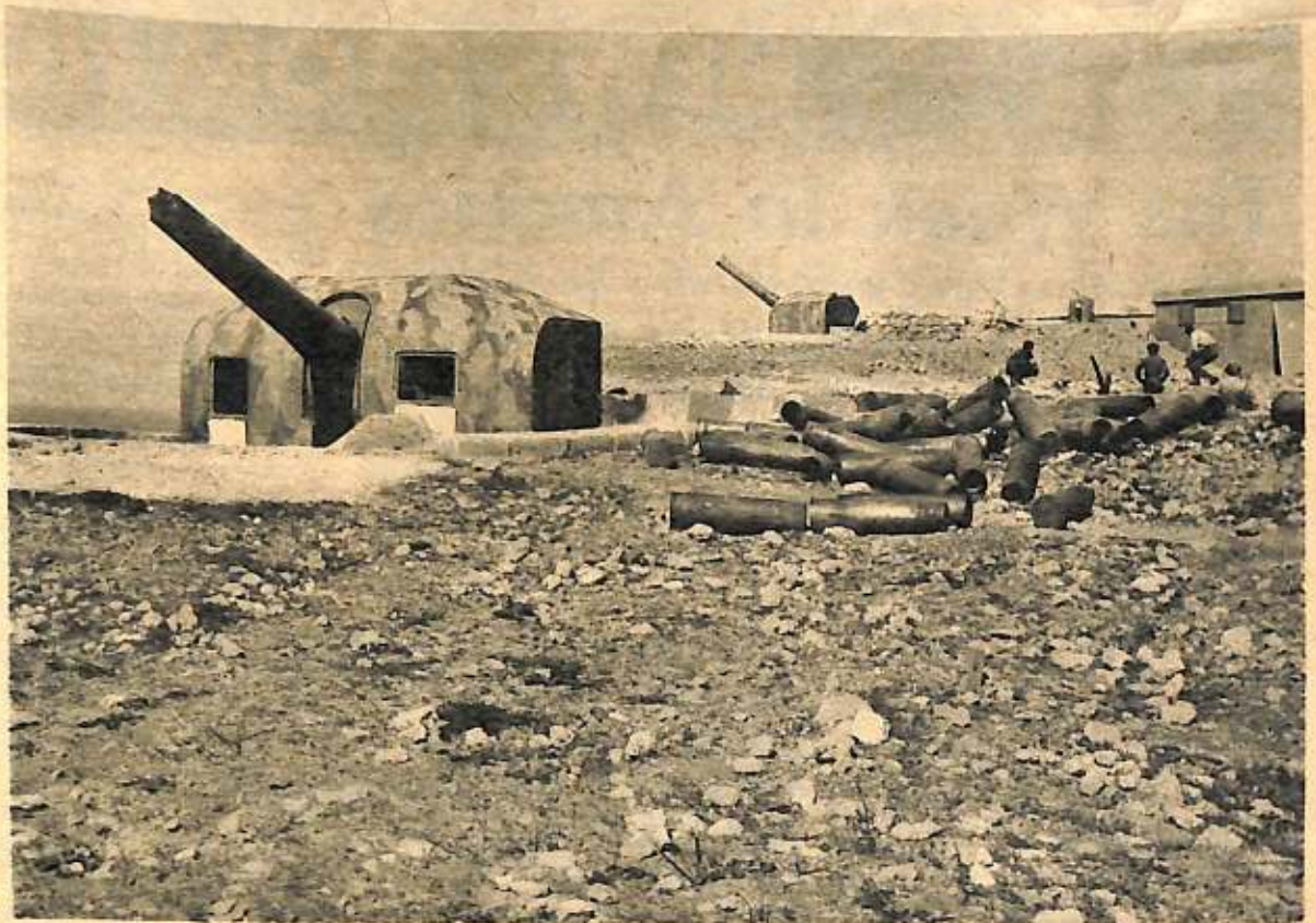
On Pointe De La Tour, Morocco; 130-mm guns were wrecked by crews, after shelling by U. S. Ships.
