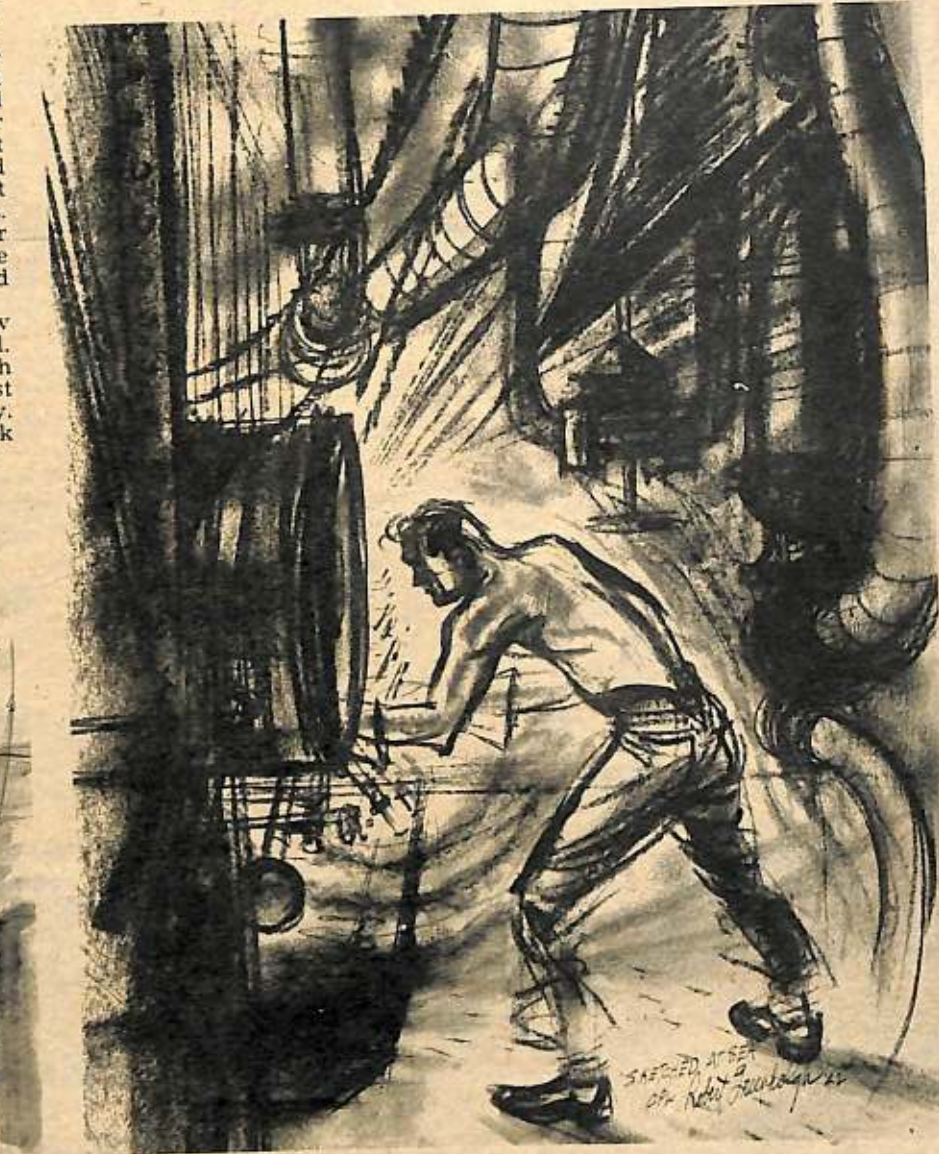
Fire room—cutting in a new burner.
