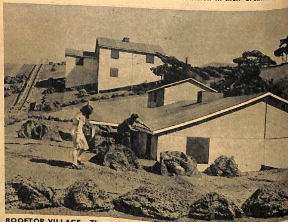
ROOFTOP VILLAGE. These are just a few of the fifty-three artificial houses built on top of Boeing's B-29 plant in Seattle to hide it from possible enemy air raids. From the sky you can't see that there are no bottom floors
