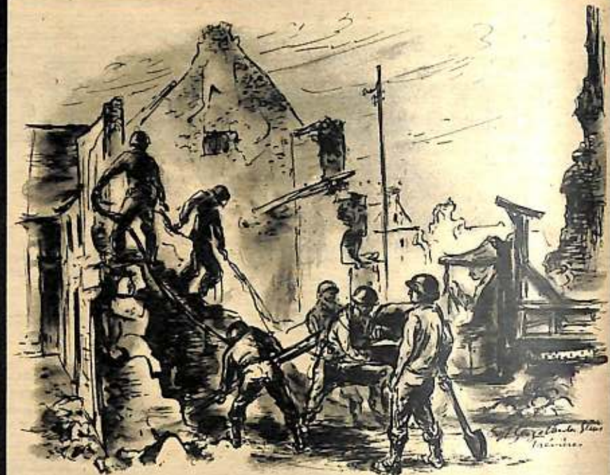
AND NOW THE ENGINEER TROOPS GET BUSY ON THE PLACE, TEARING DOWN SHELLED HOUSES AND CLEARING AWAY TONS OF DEBRIS AND RUBBLE.
