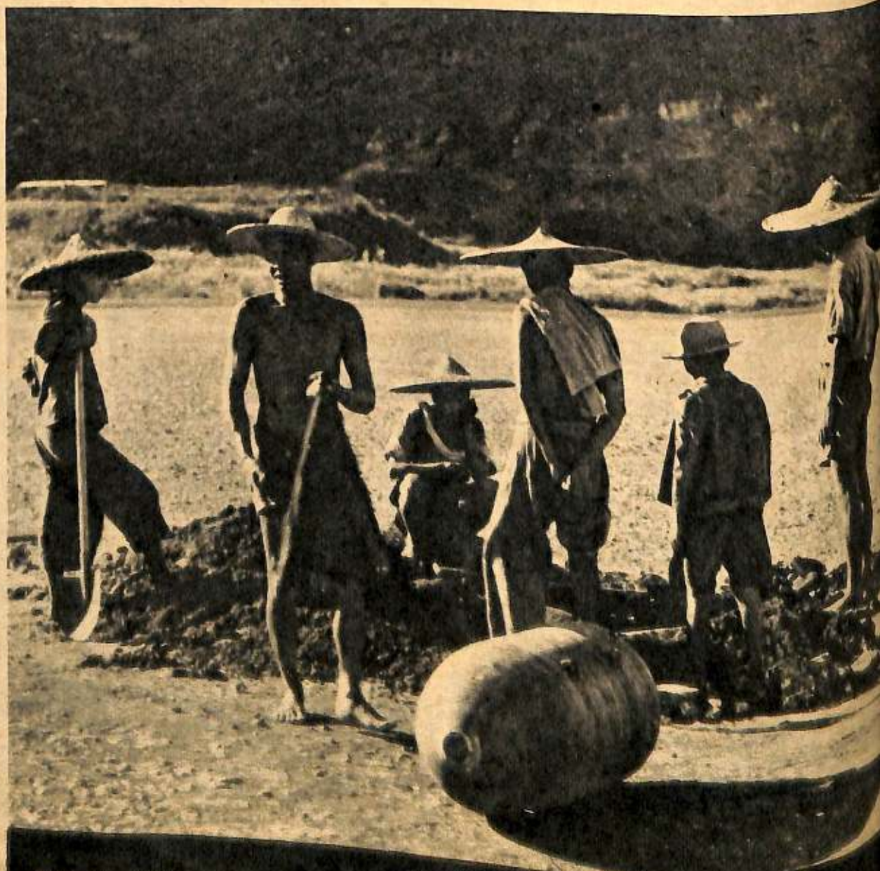
The Fourteenth Air Force takes the final step in destroying Kweilin field. They bury 1,000-pound bombs in patterns and detonate them. Craters thus formed will prevent Japs from using the base.
