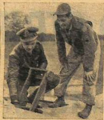
U.S. Army Air Force Photo 1/Lt. Charles F. Piche (left), of Hollis, La., and 1/Sgt. John Castro, of Key West, Fla., lower one of their ladders—designed to lessen the time spent escaping from a "ditched" Flying Fortress—into the open escape hatch above a Fort's radio room. Light and compact, the ladder can be swung into place for use within a few seconds.
