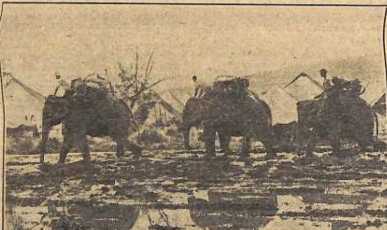
Neither rain, mud nor monsoons keeps supplies from moving forward in the CBI Theater. Superhuman endurance of natives keeps the transportation links—particularly the Burma Road—free of hazardous barriers caused by fretful nature. Top picture shows how a landslide—typical occurrence along the Burma Road—stopped a supply convoy. Chinese kids, in the center picture, are aiding their elders in clearing obstructions from the road. Pack elephants, too, pitch in with some old-fashioned plodding, but ultimately they deliver the goods.
