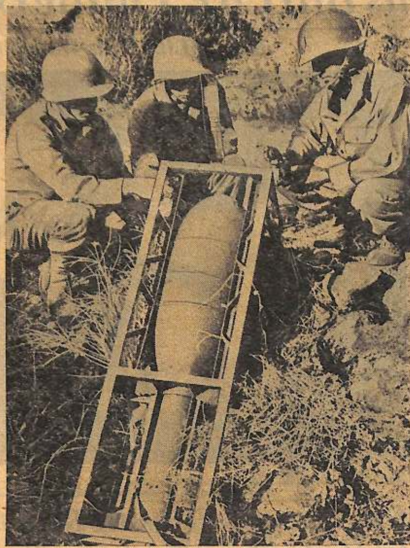
U.S. soldiers examine a German rocket captured during the campaign in Sicily. This one is known as the 32cm. incendiary rocket, and is fired directly from the crate in which it is shipped. It is seen here in firing position and takes off with a great deal of smoke and flame.
