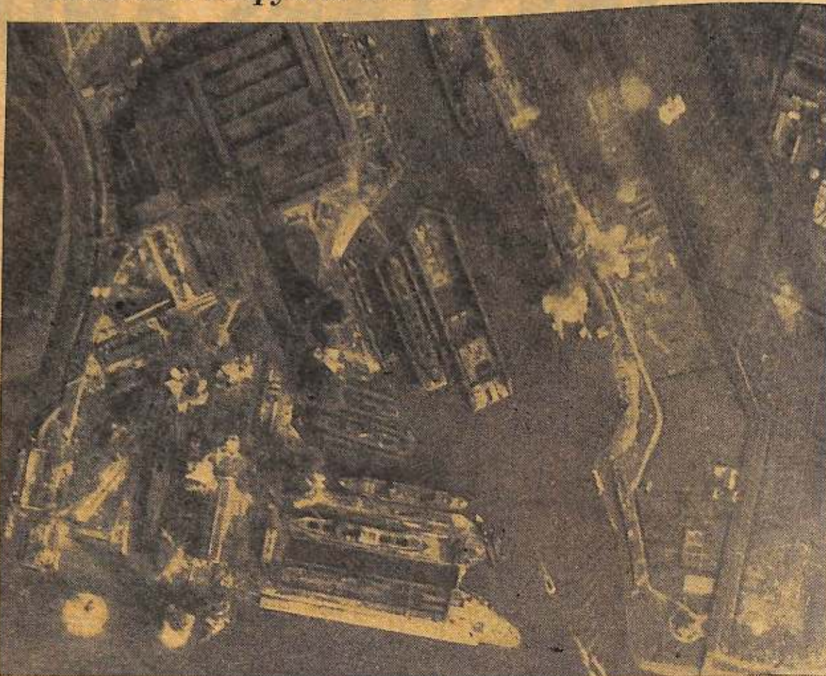
Rotterdam shipyards felt the destruction of bombs from Flying Fortresses during the successful raid Mar. 4, when direct hits were scored on ships and dock installations. This picture shows a stick of bombs exploding on submarine slips along the quayside of an engineering works.
