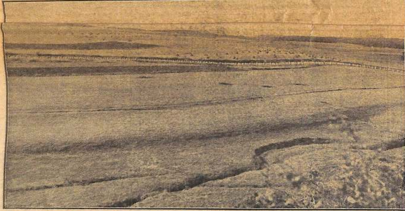
THE SIEGFRIED at long range, as Yanks up front see it. Snaking, white-dotted line is formed by concrete tank barriers, called Dragon's Teeth. Behind, barely visible in distant hills, is the objective—pillboxes.
